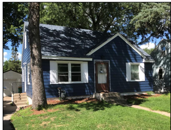
Home after using Homeowner Rehabilitation Program
