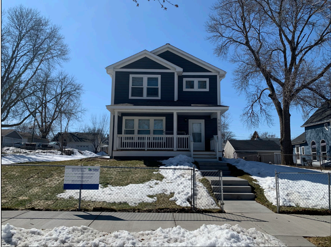
1065 Gorman Ave, constructed using HOME and NSP Funds (Photo Courtesy of Dakota County CDA)
